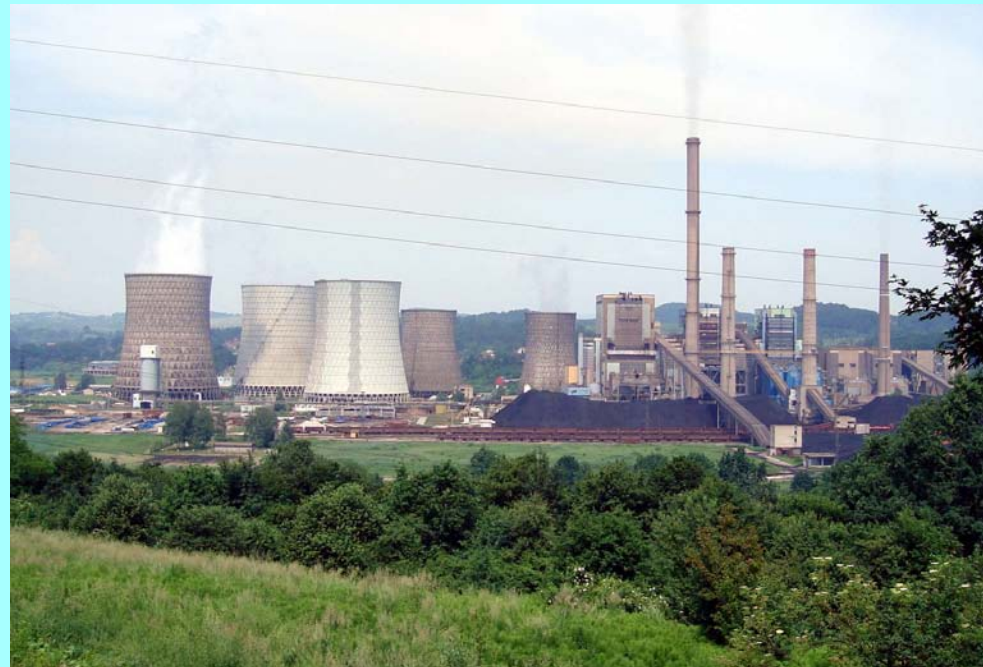
Fig.3 Open-type cooling towers in "Tuzla" Power Plant
